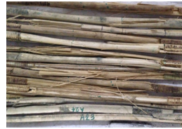
(b) Failure Pattern
